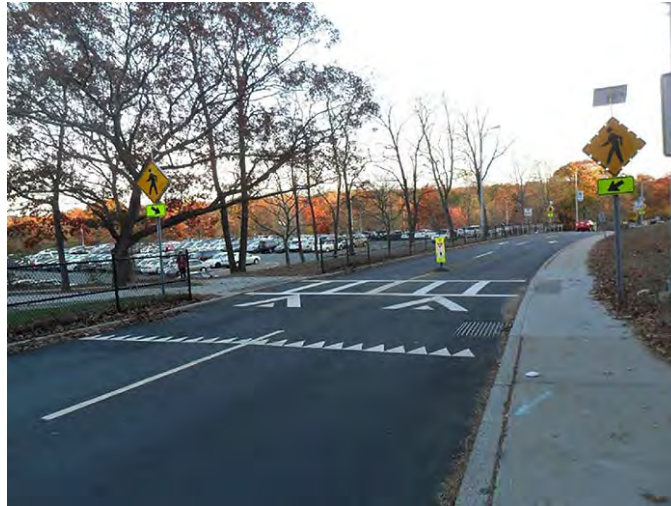
Figure 9: Raised Crosswalk Example
